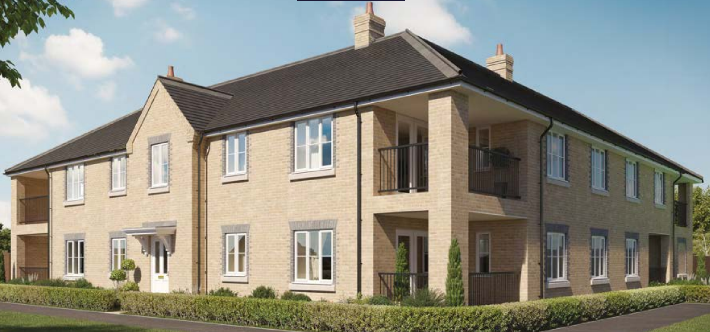
The Maypole Apartments
